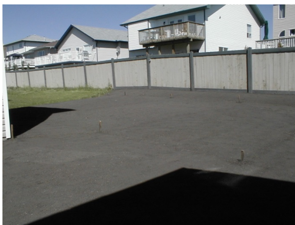
Internal swale at final grade stage (with string lines as a guide) directs surface water towards the side common property swale.
