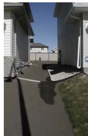
Good final grade drains water in the common swale
