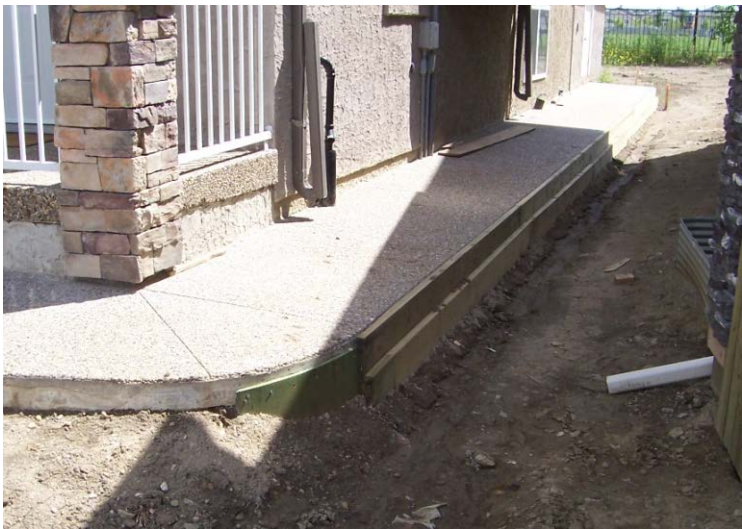
A sidewalk must allow 15 cm from the property line for a drainage swale
