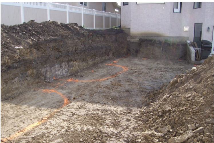
A retaining wall location is marked on the ground and will be built to control the surface drainage in this 'walk-out' development
