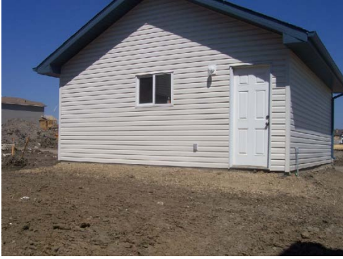
This is good grading with slope away from the detached garage
