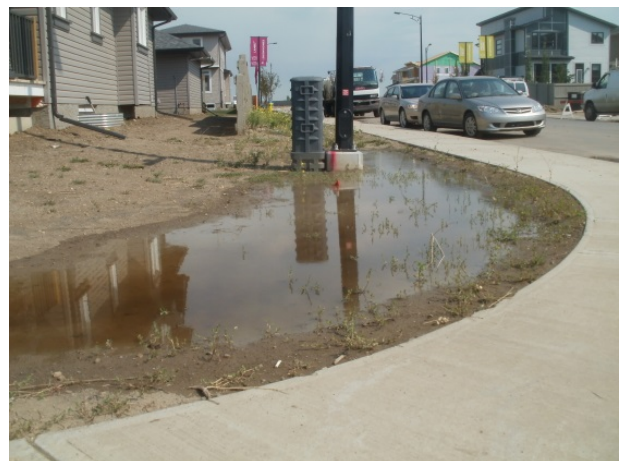
Clay cap is graded at Rough Grade Stage to meet the requirement for interim pooling behind the public sidewalk / curb
