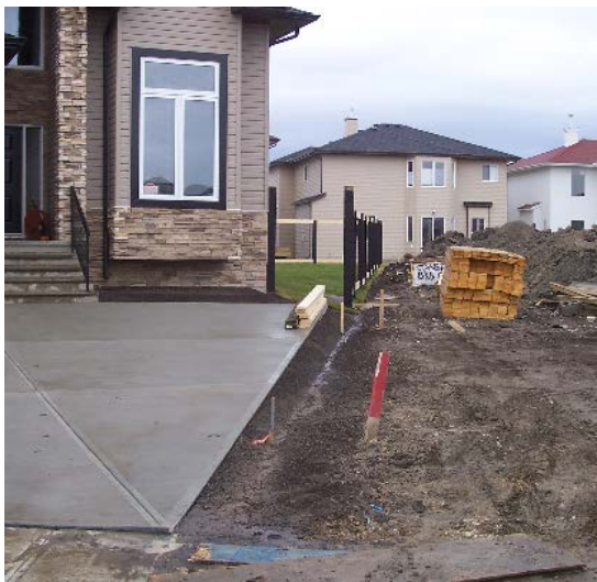
Driveway built 15 cm from the property line for common swale
