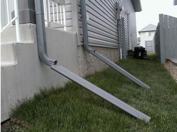
Downspouts with extensions direct water to swale
