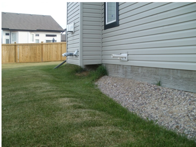
Settlement creates negative grade towards the foundation and can lead to drainage problems
