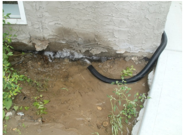
Re-circulation of ground water due to settlement and sump pump hose location
