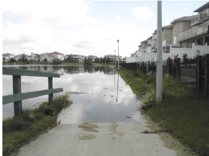
Walkways are flooded after rain events, as designed, to manage stormwater
