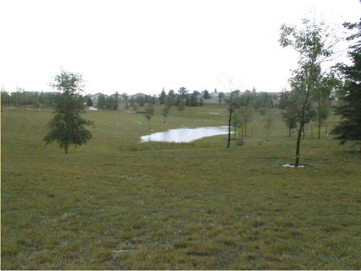
Dry-pond recreation areas accumulate stormwater during rain events to control water volumes flowing into the storm sewer system
