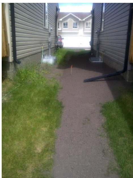
Grading repairs for settlement at foundation walls and property line swale will be needed however, consultation with adjacent owners is advised to avoid problems
