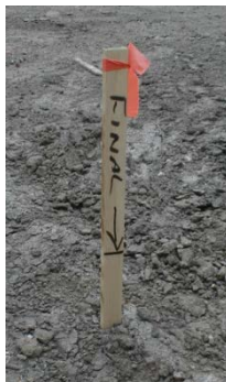
Grade stakes indicate the off-set and the design elevations for topsoil
