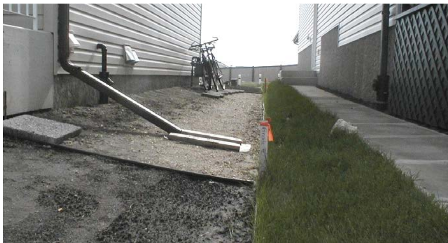
This rough grade base has been raised to match the final grade before placing decorative rock. Ponding will be minimized or eliminated
