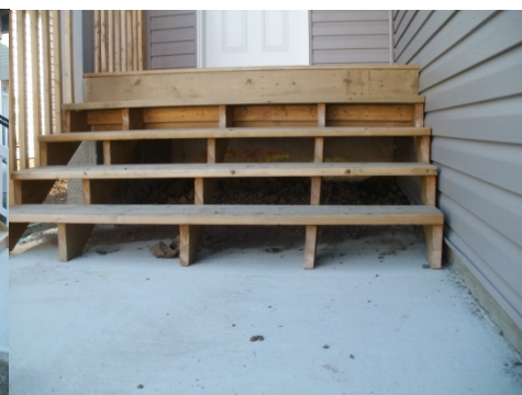
Backfill under a front step
