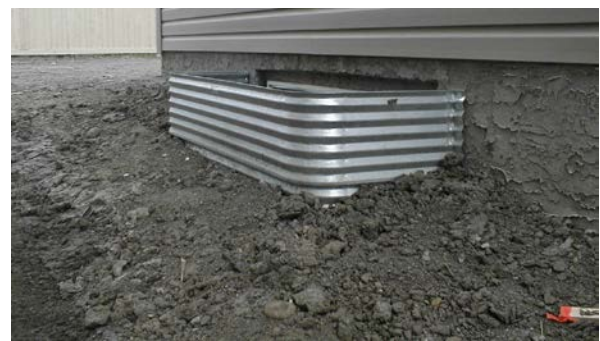
Positive grade away from foundation at window well
