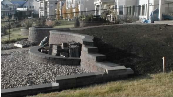
These retaining walls are built within the easement
