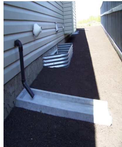
The splash pad conveys water from the sump pump discharge pipe past the foundation excavation zone
