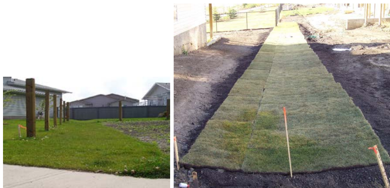
Registered easements or right-of-ways allow for concrete or grass drainage swales on private property
