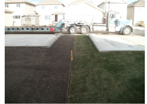
Garage pads (at rough and final grade stages) have been built with retaining walls for future garages
