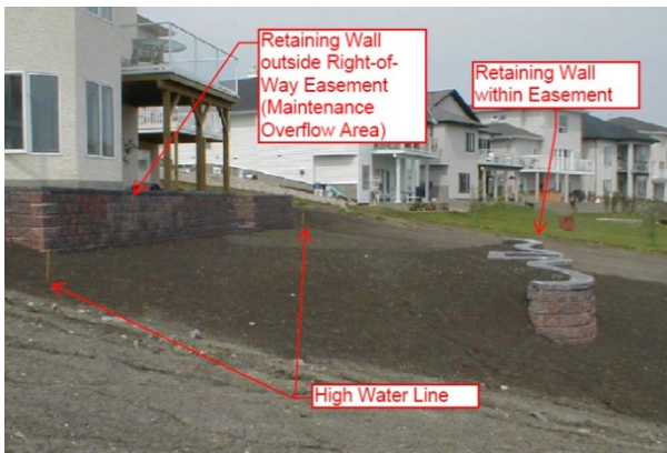
Retaining walls are built inside and outside the Easement
