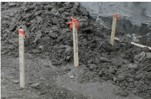
Grade stakes indicate the off-set and the design elevations for topsoil
