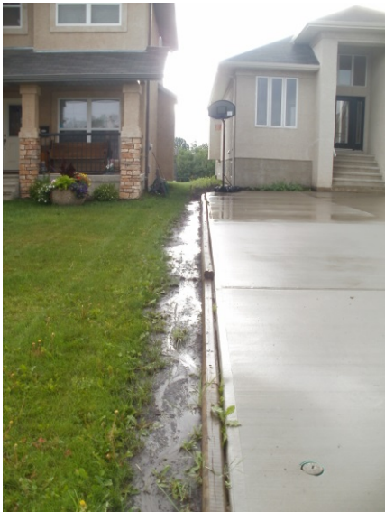
Retaining wall at driveway reduces steepness to the common swale
