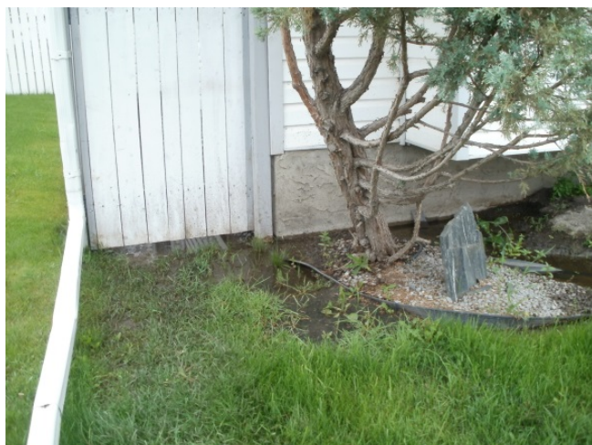
Settlement creates negative grade towards the foundation and can lead to drainage problems
