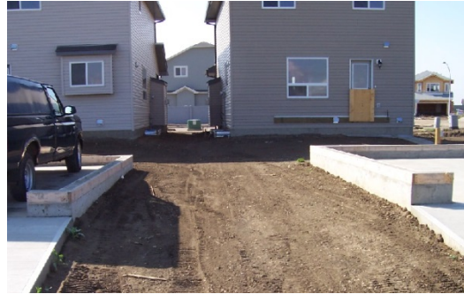
Garage pads (at rough and final grade stages) have been built with retaining walls for future garages
