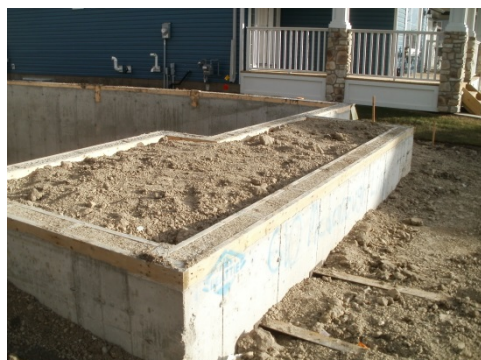
Pre-grading backfill for a future front deck
