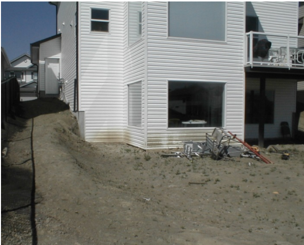
Rough grade is prepared for future retaining wall construction
