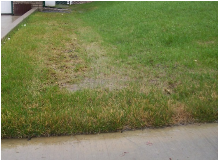
Settlement on drainage swales should be repaired
