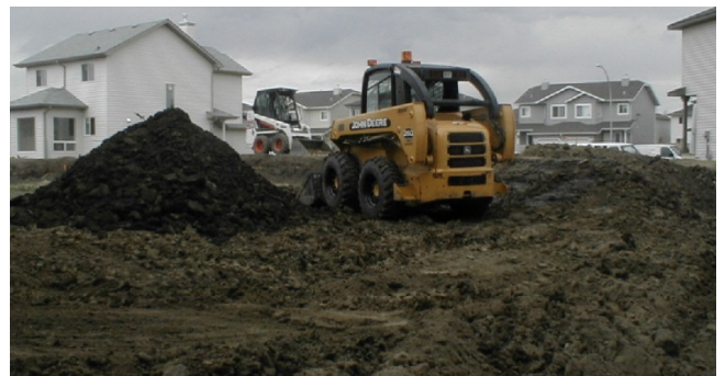
Grading in progress at rough grade stage
