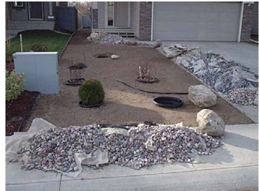
Compacted road-crush gravel, set to final grade, directs water over the sidewalk to the street
