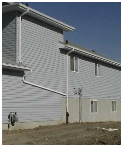
Typical connections for downspouts to storm service
