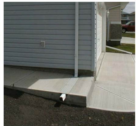
Downspout with extension under concrete
