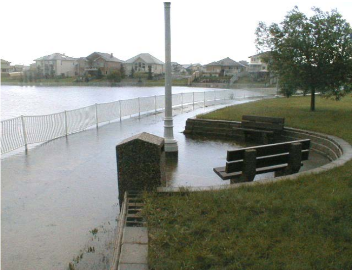
Walkways are flooded after rain events, as designed, to manage stormwater
