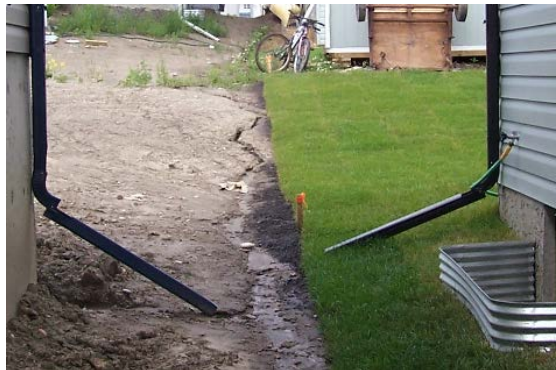
Downspout extensions discharge water to the swale at the common property line
