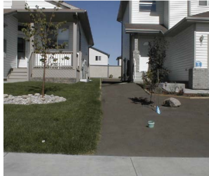
Sod and topsoil at final grade stage
