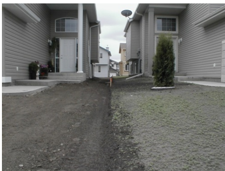
A common swale between rough and final grade stages
