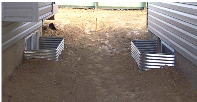
Rough grading slopes towards the common drainage swale
