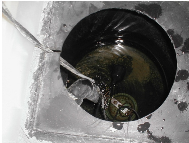
Typical residential sump-well with installed sump pump
