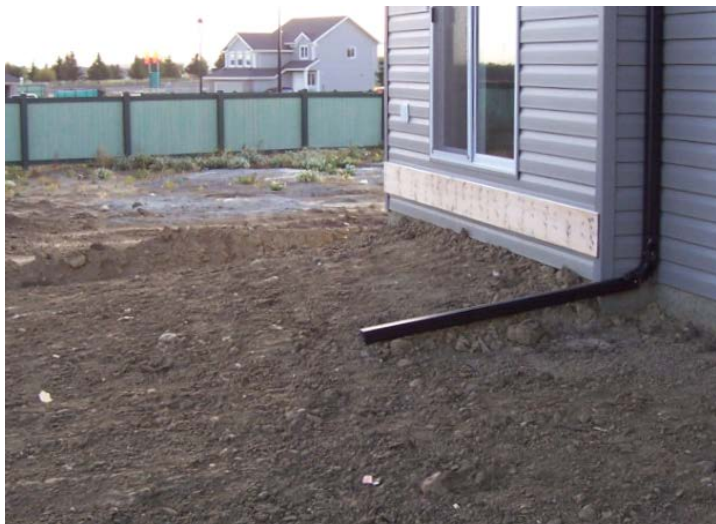
Slope away from the foundation wall below a future deck
