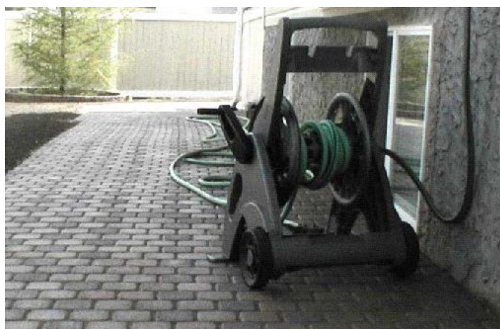
A decorative hard surface at 0.75% minimum slope
