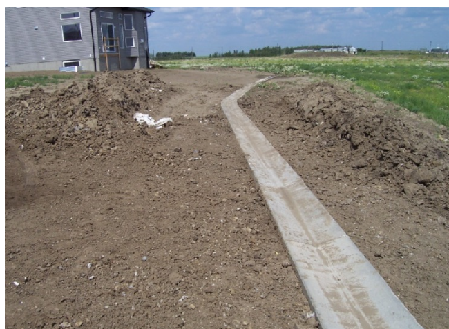
Concrete swale in drainage easement or right-of-way
