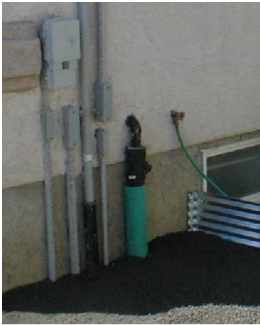
Sump pump is connected to foundation service
