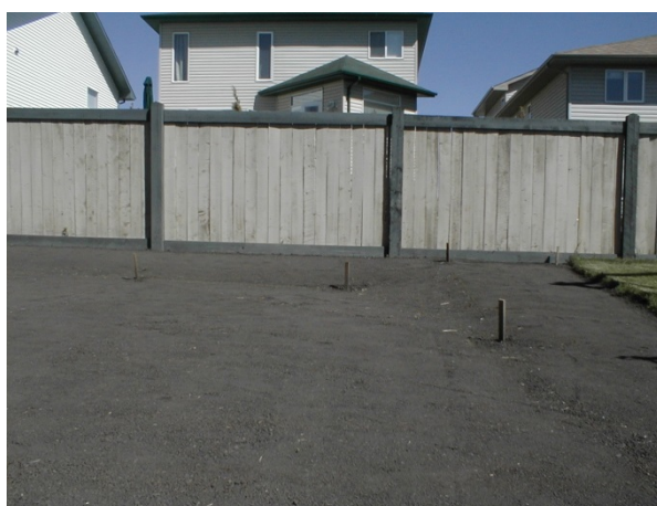
Internal swale at final grade stage (with string lines as a guide) directs surface water towards the side common property swale.
