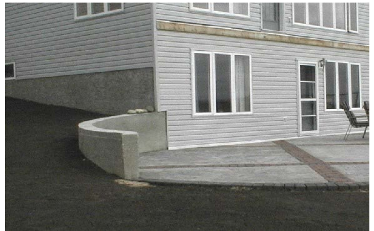
A retaining wall attached to the walk-out basement
