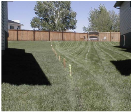
A string-line is used as a guide for the grass swale which has a minimum of 1.5% slope
