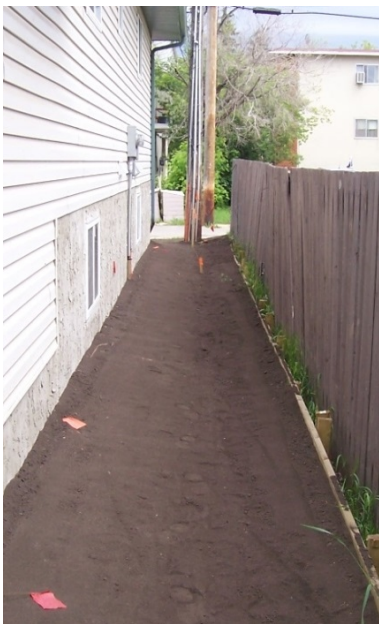
An internal swale is graded with topsoil and an independent retaining edge
