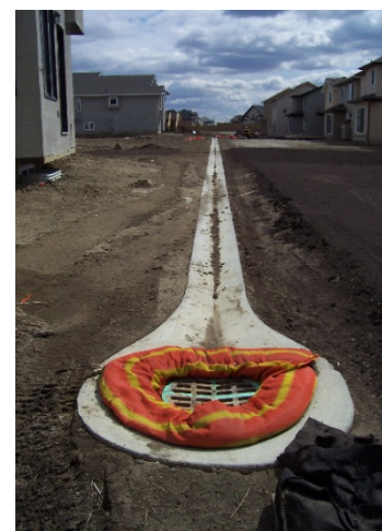
Concrete swale with a catch basin and temporary sediment control
