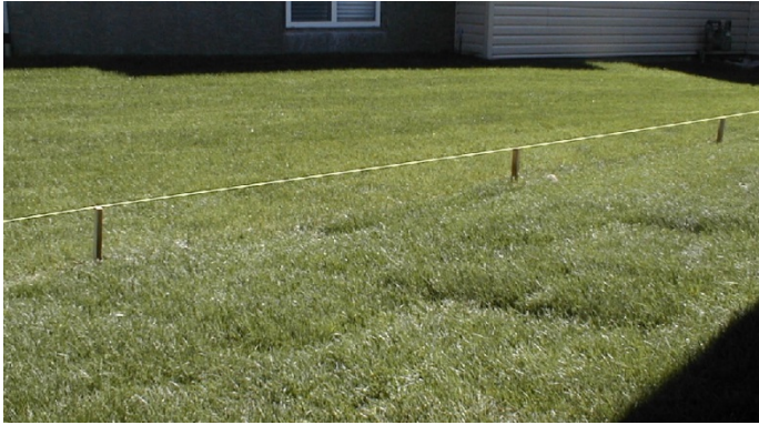
A string-line is used as a guide for the grass swale which has a minimum of 1.5% slope
