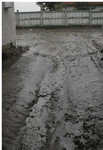
Swale conveys water during heavy rain
