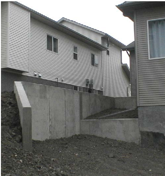
A retaining wall has been built to control surface drainage at this 'walk-out' development
