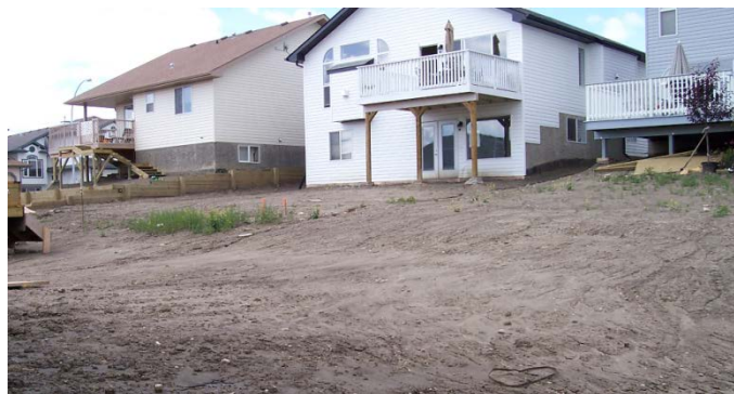
Lot-to-lot drainage occurs due to the topography
