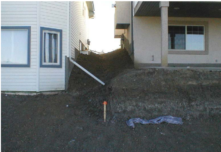
These lots have a large grade differential at the common drainage swale
