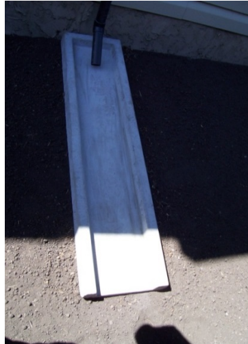
The splash pad conveys water from the sump pump discharge pipe past the foundation excavation zone
