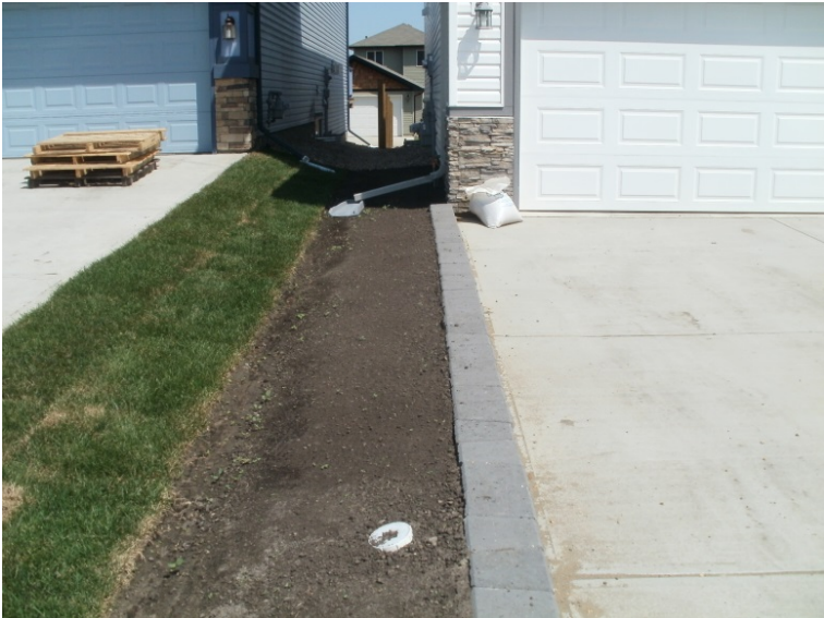
Retaining wall at driveway to control cross-lot drainage
