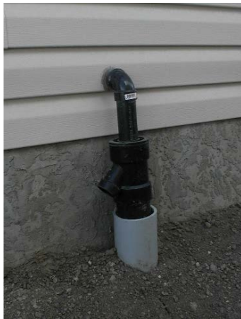
Sump pump discharge pipe is connected to the foundation service
