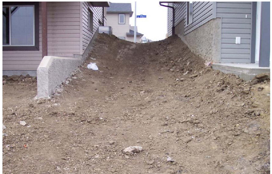
A retaining wall on one side supports the common property swale between these two 'walk-out' developments
