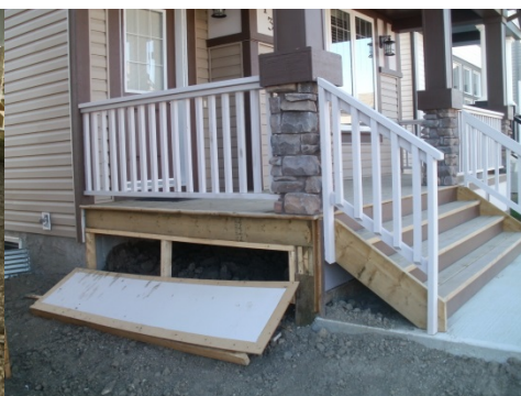
Exterior deck skirting removed to backfill under a front deck
