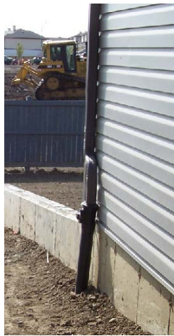
Typical connections for downspouts to storm service
