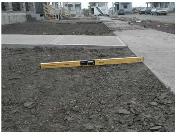
Clay cap is graded at Rough Grade Stage to meet the requirement for interim pooling behind the public sidewalk / curb
