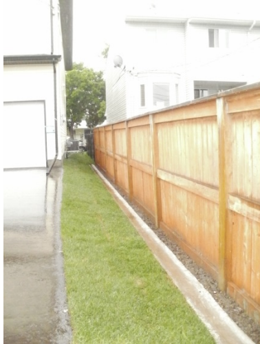
Internal side-lot swales with retaining walls that are independent of the common property fences
