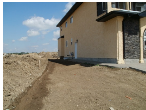
A rough grade swale adjacent to an undeveloped lot.
