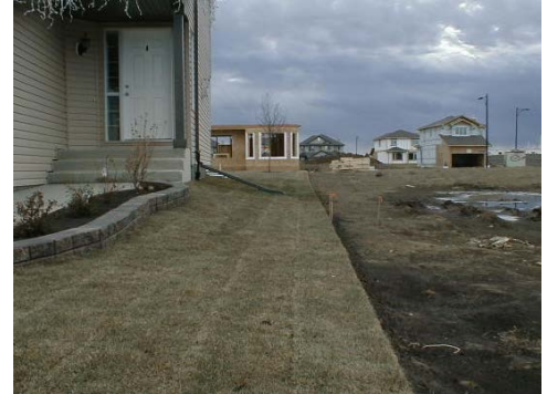
Final grade stage adjacent to an undeveloped lot
