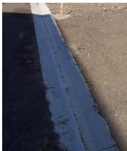
Concrete swale in drainage easement or right-of-way
