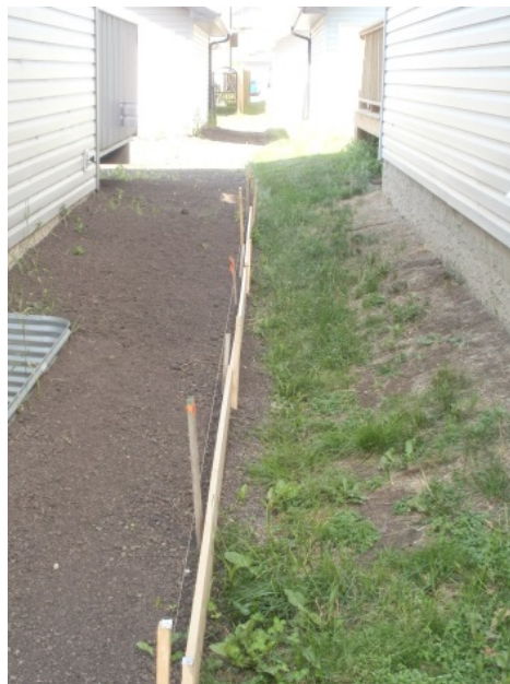
Grading repairs for settlement at foundation walls and property line swale will be needed however, consultation with adjacent owners is advised to avoid problems
