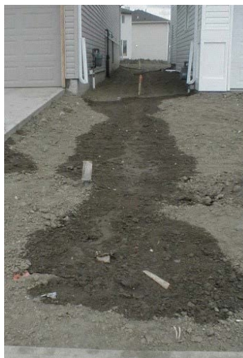
A light rain proves that the swale drains properly
