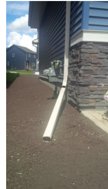
Downspout extensions discharge water to the swale at the common property line
