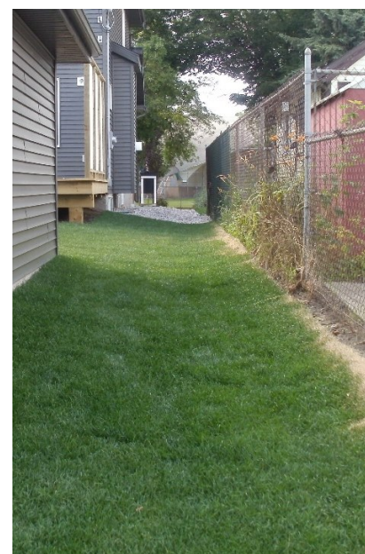
An internal swale with sod
