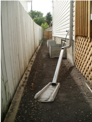
Internal side-lot swales with retaining walls that are independent of the common property fences
