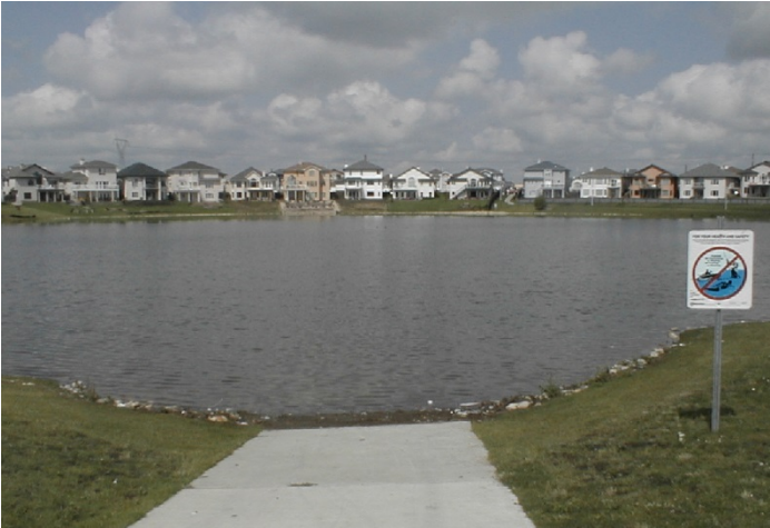
A stormwater management lake at normal water level. Sign shows the location of the designed high water level
