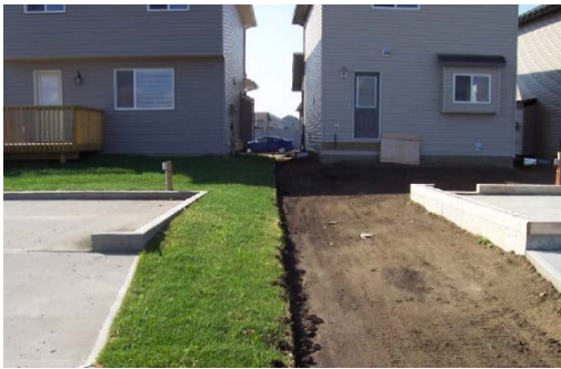
Garage pads (at rough and final grade stages) have been built with retaining walls for future garages
