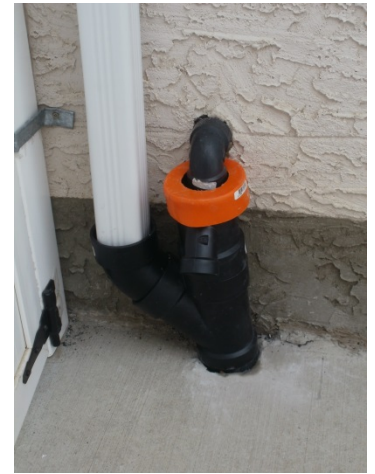
Downspout and sump pump are connected to storm service
