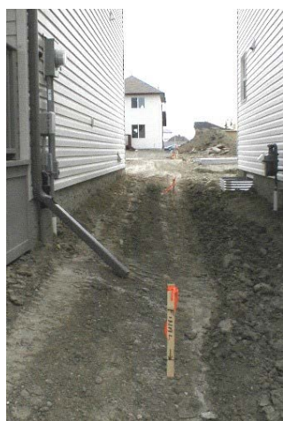
Rough grade drains water away from the wall
