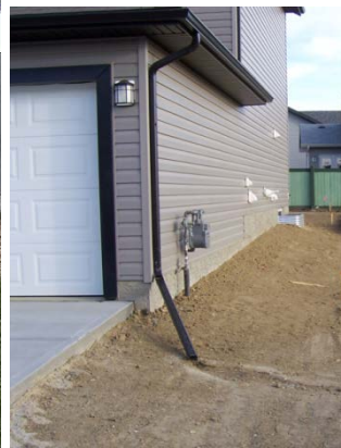
Downspouts with extensions direct water to swale
