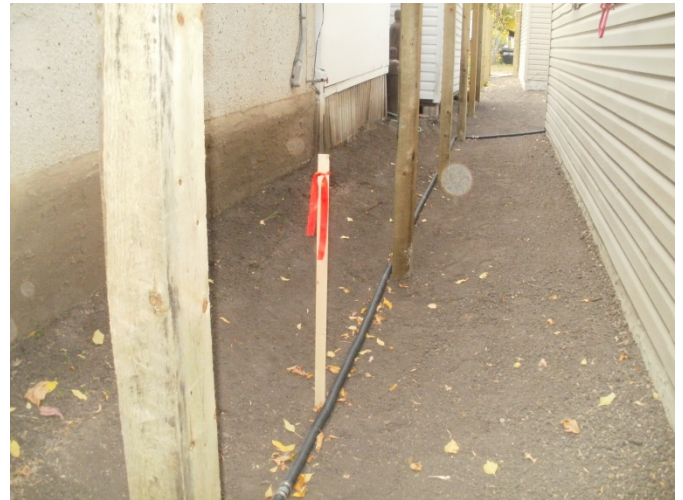
A common swale created when neighbouring owners work together
