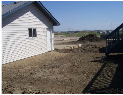
An internal swale is built between the detached garage and the house
